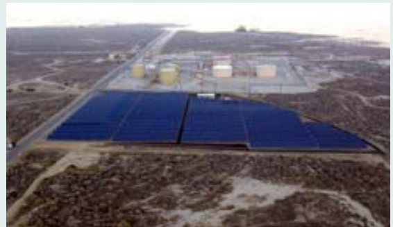
United Solar Ovonic thin-film solar cell technology is being commercialized on five continents — in everything from residential roofs, to bottling plants, to augmenting power to a six-acre oil field in California.
